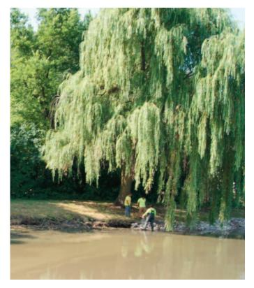
This photo shows Wilderness Pond South shoreline being lined with rip rap by Fremont Township Highway staff. Observe the significant erosion and sediment suspended in the water. This shoreline was repaired in 2018 during this SMC WMB grant by Fremont Township and MPRD to help prevent sediment flowing into Diamond Lake. Photo by Tori Trauscht.
